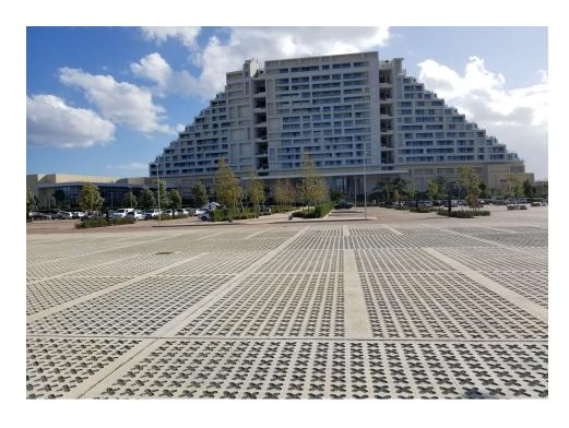
Constructing this massively impressive hotel and casino resort, called for radical solution to its car parking requirements, with in particular the casino likely to create an intensive use, when compared to the normal visitor/parking ratios of more traditional hotels. A significant factor in the design was the need to introduce an effective surface water control system, without a requirement for major changes to the drainage infrastructure and local eco-system.
