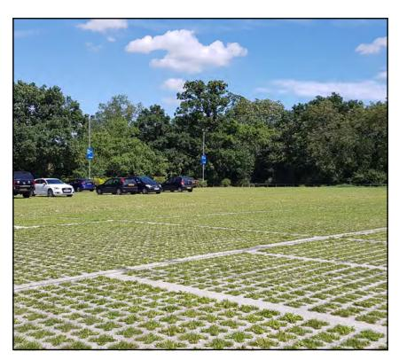
The first phase of this stadium redevelopment, undertaken in 2016, featured a 5600 m<sup>2</sup> spectator car park, constructed from 76mm thick Grasscrete GC3 paving, but within which there was an access link to a future extension. This was constructed from 150mm thick Grasscrete GC2, so as to enable access for construction traffic to those works.
