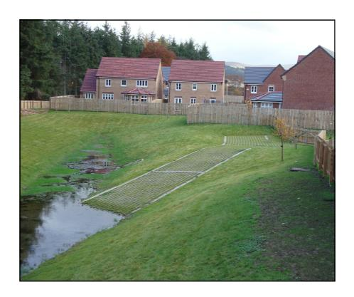
The focus on storm water management in the UK is steadily shifting away from traditional piped sewers to surface attenuation as shown here with this housing project. By retaining storm water on site the peak demand on the main sewer infrastructure has been reduced and a landscaping amenity gained.
