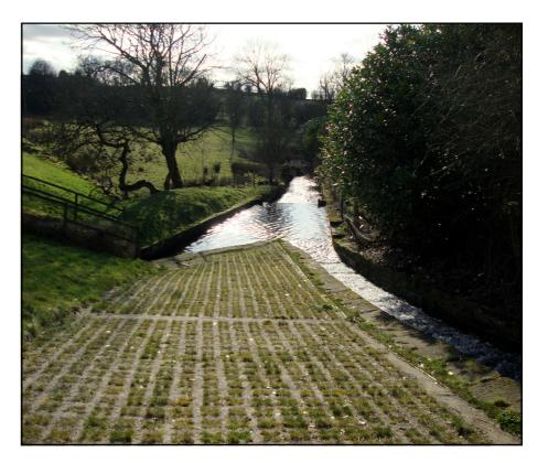
Mature reservoir projects can pose a challenge to contractors called in to undertake upgrading works. The site and the available access may no longer resemble what was available to the original builder. This was the case for this project, where a Reservoir Inspection had identified the need to armour the ground around and between its overflow and by-wash channels.
