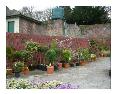
There's perhaps no better place to showcase a plantable retaining wall than by constructing one within the grounds of a popular new garden centre. For this project in Cumbria the large open air display area called for a significant earthworks cut with a resulting need to retain the surrounding ground as well as introducing buttressing to a number of structures.
